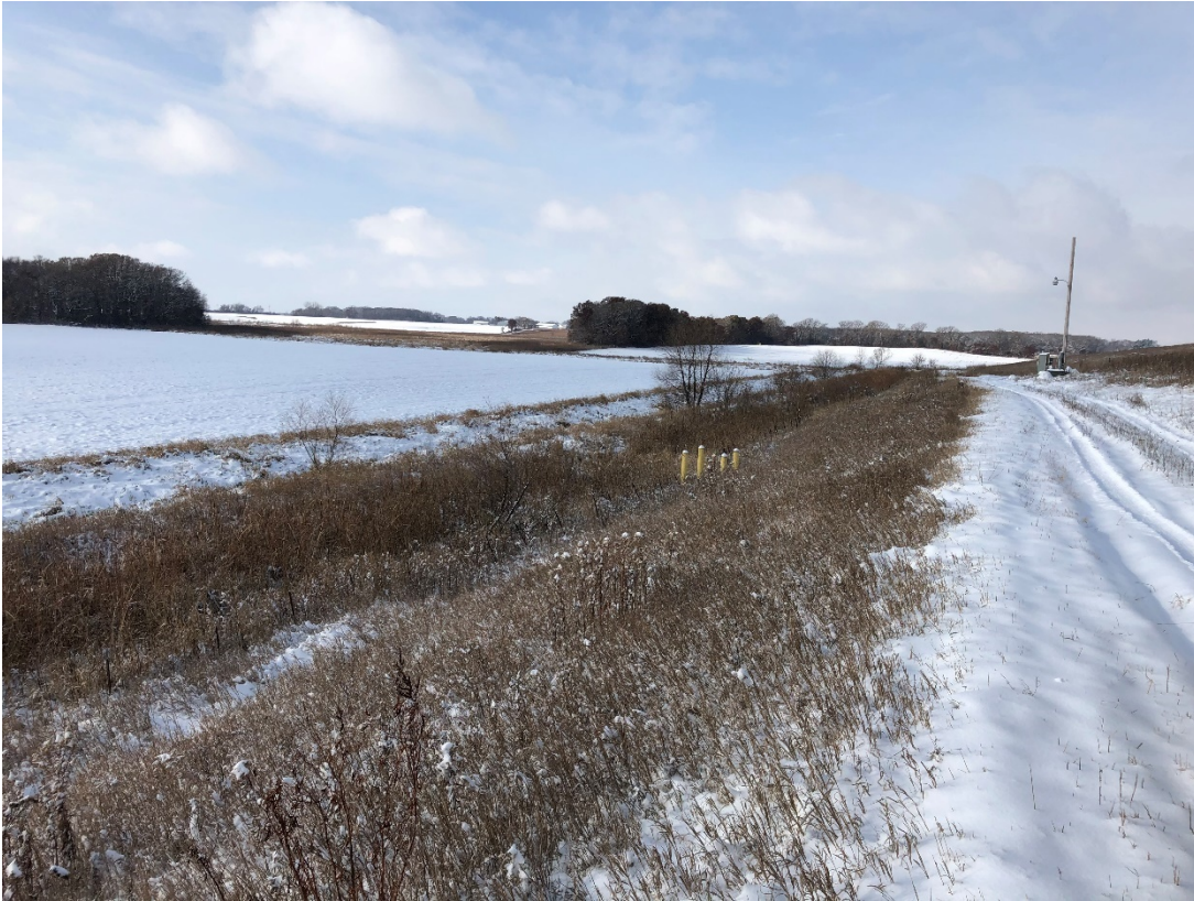
Photo 17: Location 7 – Looking West, Phase 2 Southern Berm
