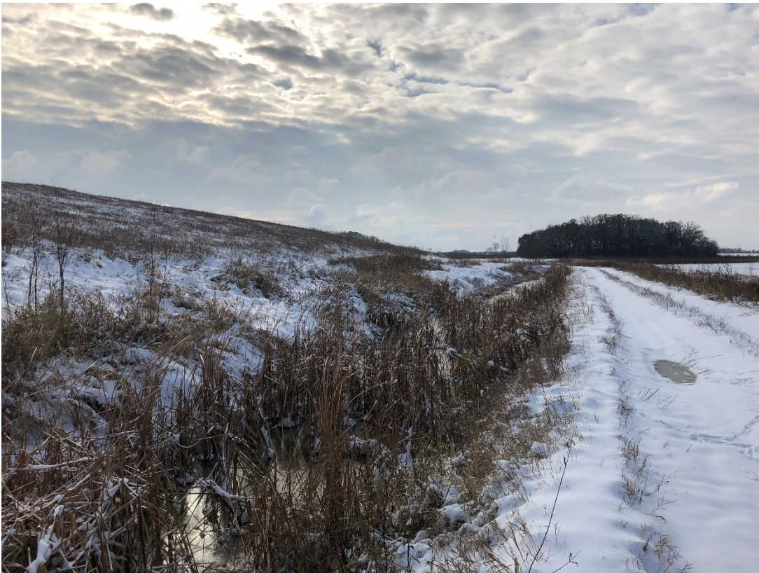
Photo 6: Location 3 – Looking South, Toe of Phase 1 Western Slope
