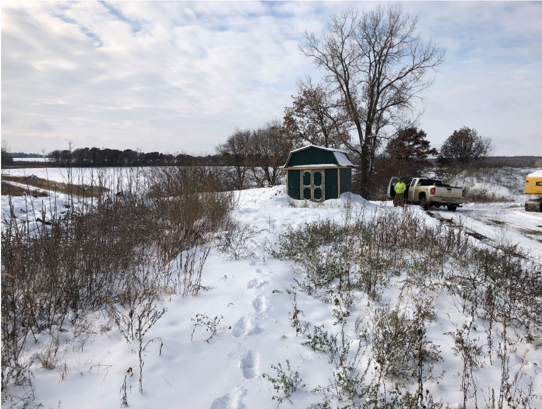
Photo 3: Location 1 – Looking Southwest, Phase 4 Anchor Trench
