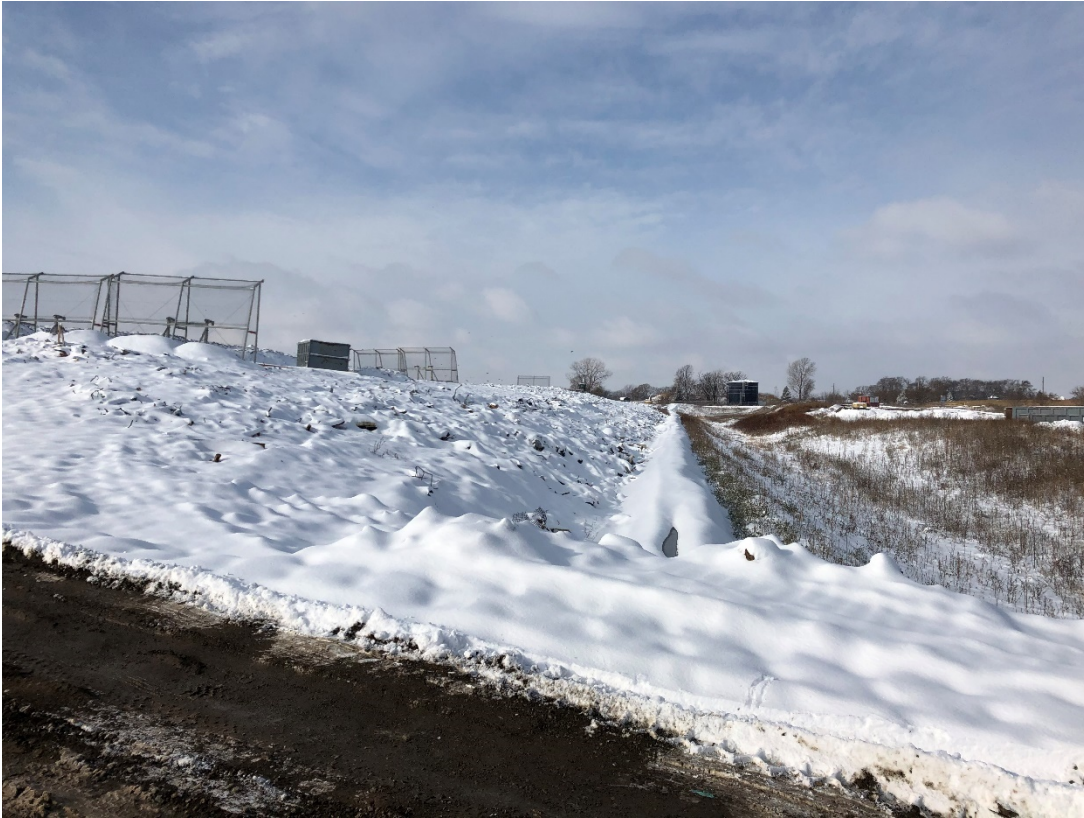
Photo 33: Location 12 – Looking West, Phase 4 Northern Rain Flap
