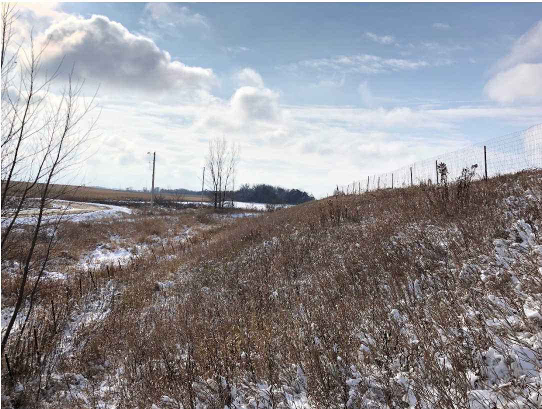
Photo 26: Location 9 – Looking South, Phase 2 Eastern Berm
