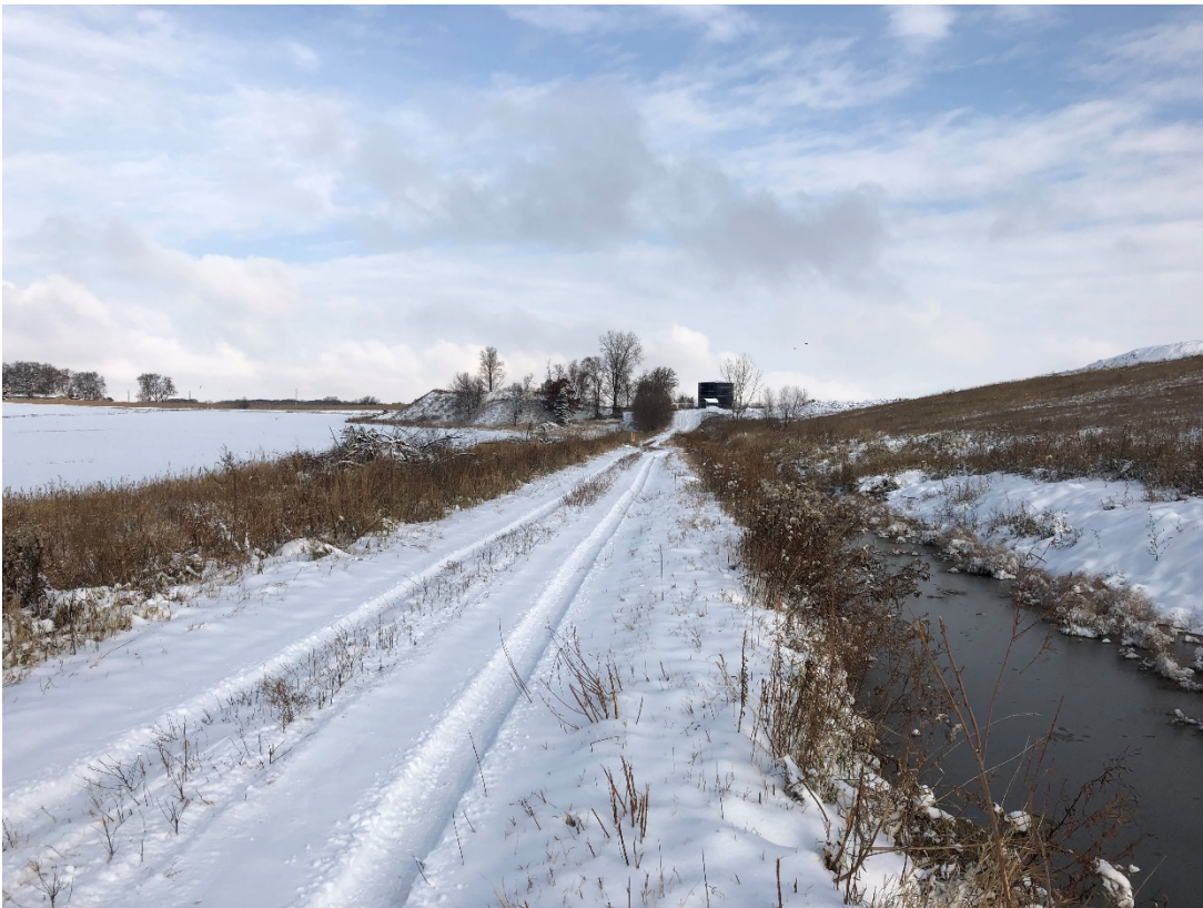
Photo 8: Location 4 – Looking North, Toe of Phase 1 Western Slope
