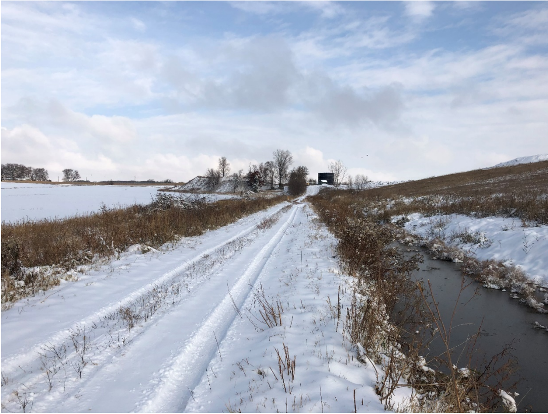
Photo 7: Location 3 – Looking North, Toe of Phase 1 Western Slope
