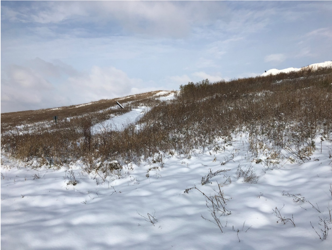
Photo 13: Location 6 – Looking West, Phase 1/2 Overlay Liner & Southern Slope
