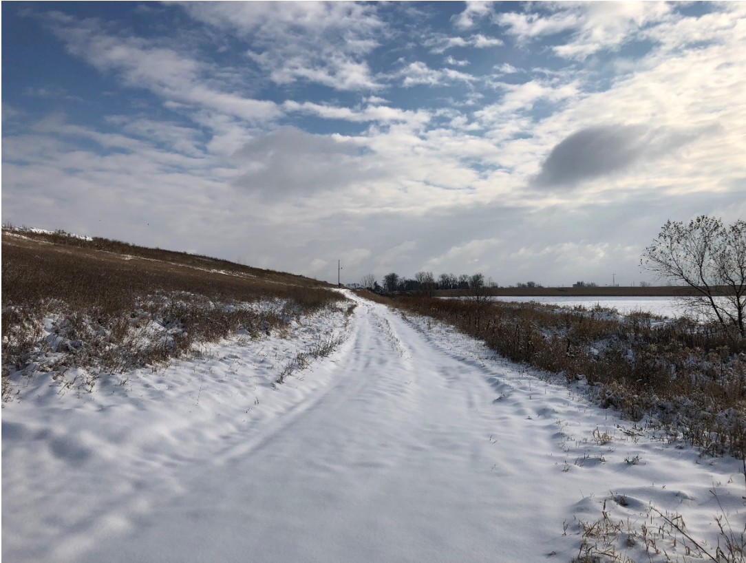
Photo 9: Location 4 – Looking East, Toe of Phase 1 Southern Slope
