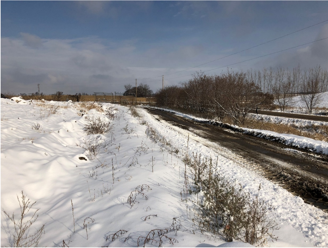
Photo 31: Location 11 – Looking North, Phase 4 Eastern Anchor Trench
