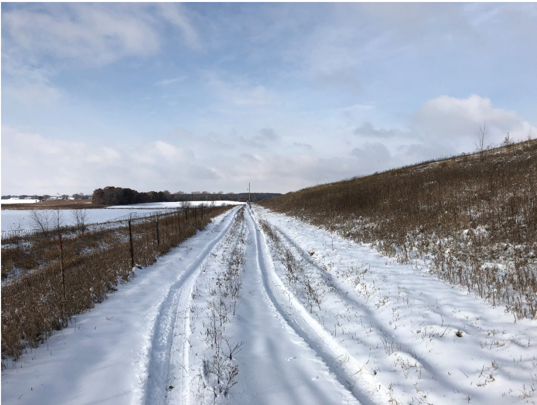
Photo 20: Location 8 – Looking West, Phase 2 Southern Perimeter Road and Slope
