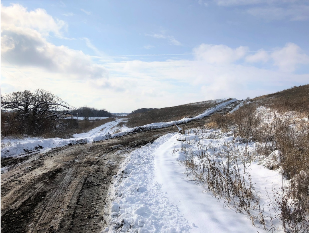
Photo 29: Location 10 – Looking South, Phase 2 Eastern Slope and Interior Access Road Entrance
