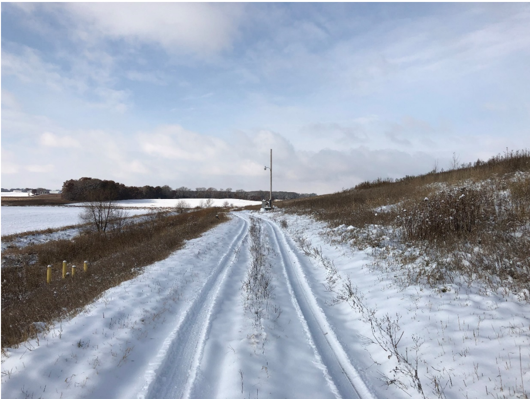
Photo 16: Location 7 – Looking West, Phase 2 Southern Perimeter Road and Slope
