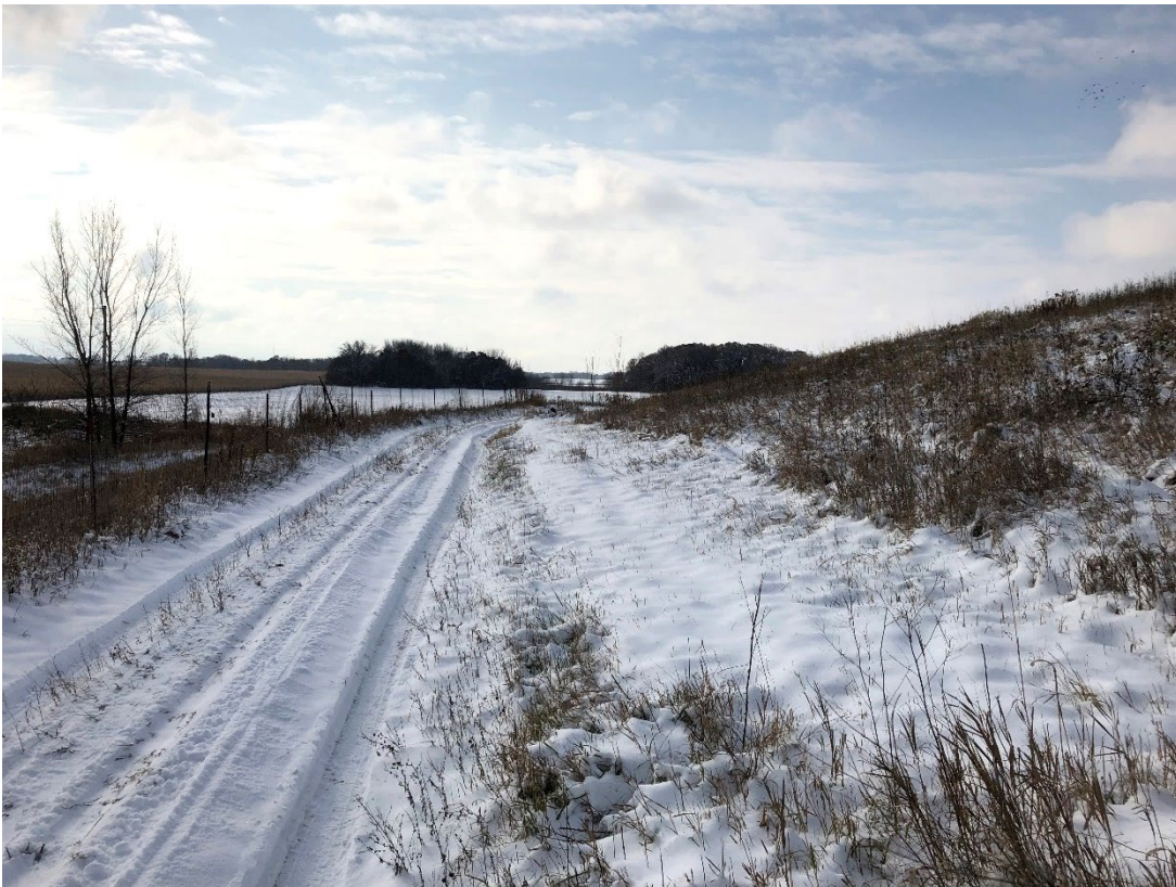
Photo 24: Location 9 – Looking South, Phase 2 Eastern Perimeter Road & Slope
