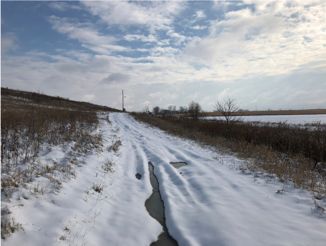
Photo 11: Location 5 – Looking East, Toe of Phase 1 Southern Slope
