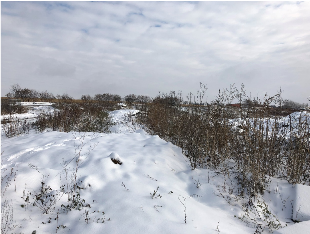
Photo 4: Location 2 – Looking Northeast, Phase 4 Anchor Trench
